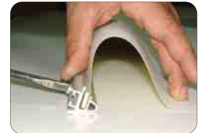
Place the pressure bar fully into the rail and tighten screws
