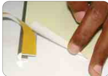
Register the graphic with the top edge of the rail Remove the release liner slowly
